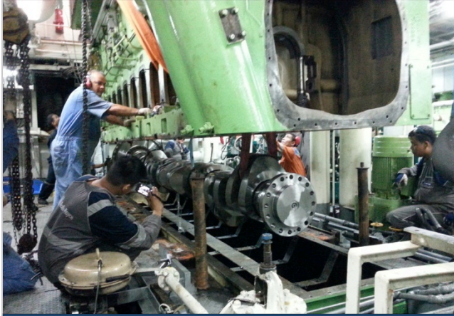
Crankshaft installation in process
