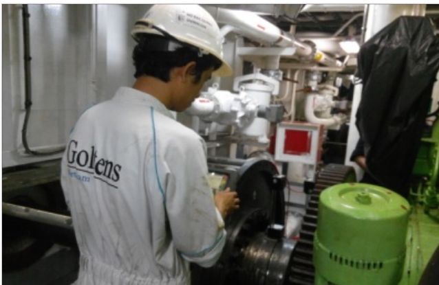
Laser Alignment of engine
