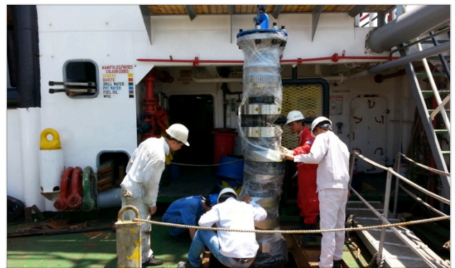
Rigging of replacement crankshaft onboard
