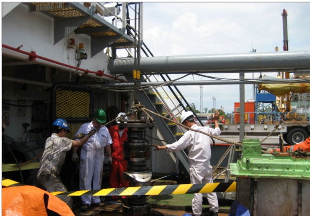
Rigging condemned crankshaft off vessel
