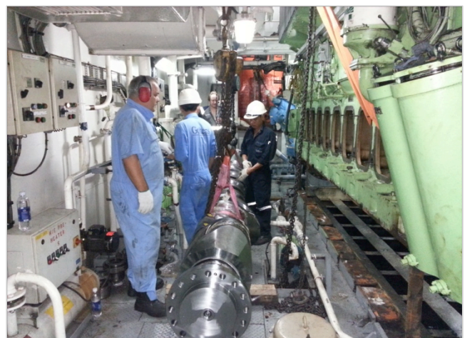
New crankshaft on deck in engine room
