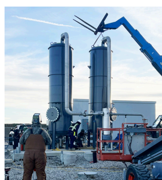
PRESSURE-TESTING OF THE ENTIRE SYSTEM
