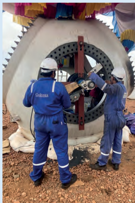
Machining the two-step inner diameter of the WTG hub to required dimensions
