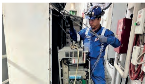
Installation of overhauled VFD
