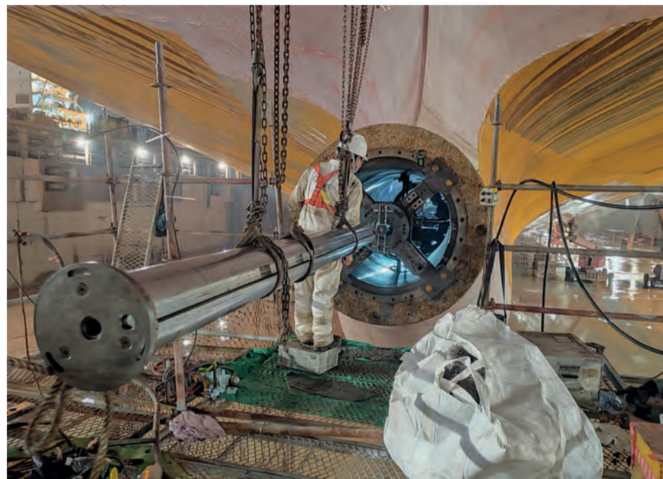
In-situ line boring of stern tube housing
