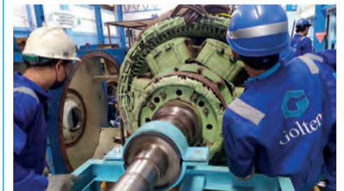
Removal of the stator from generator
