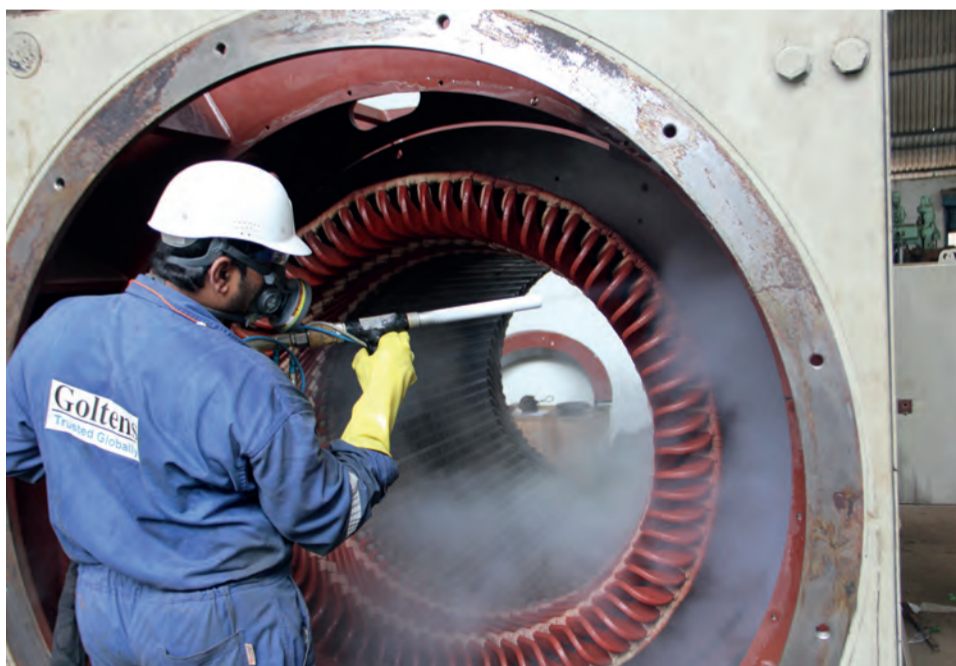
CO2 Cleaning of generator stator
