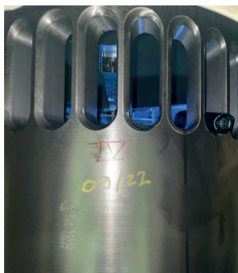
LDM equipment installed on top of the Liner
