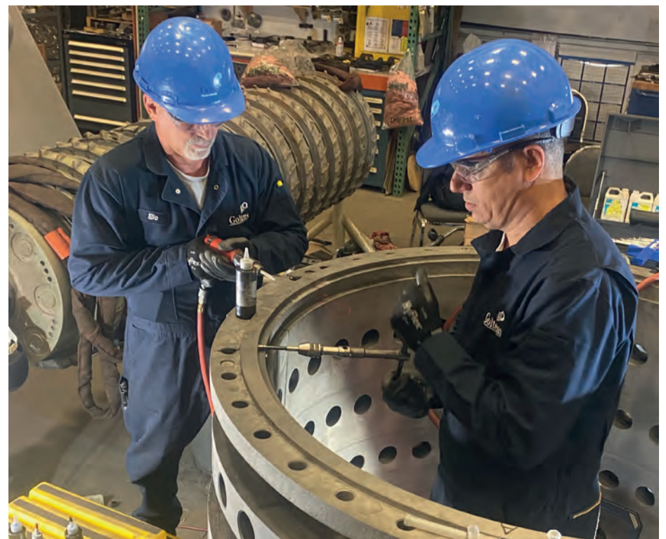
Tapping drilled holes along crack for stitching pins
