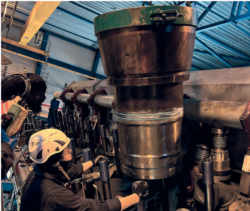
Goltens' technician removing cylinder liner from engine
