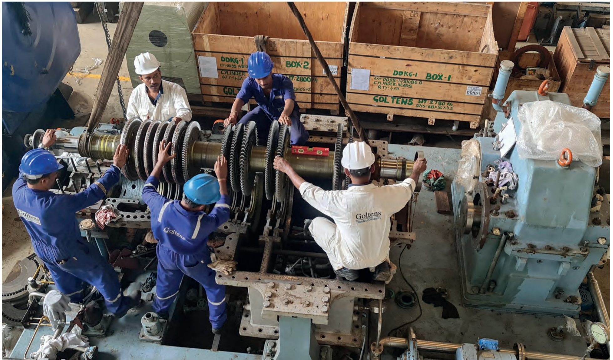
Performance of clearance checks on rotor placement
