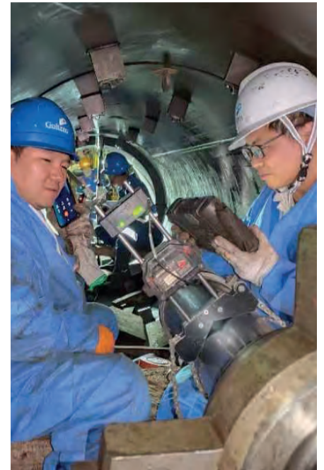
Laser alignment of in-situ boring equipment
