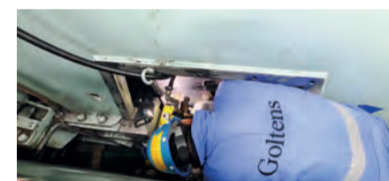
Tools and technician working in highly confined space with limited clearance
