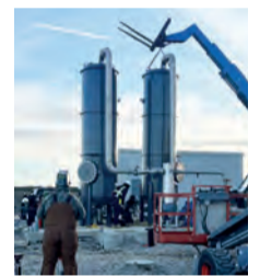
Pressure-testing of the entire system
