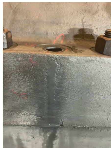
Stitching pins installed, surface dressed prior to metal lock installation
