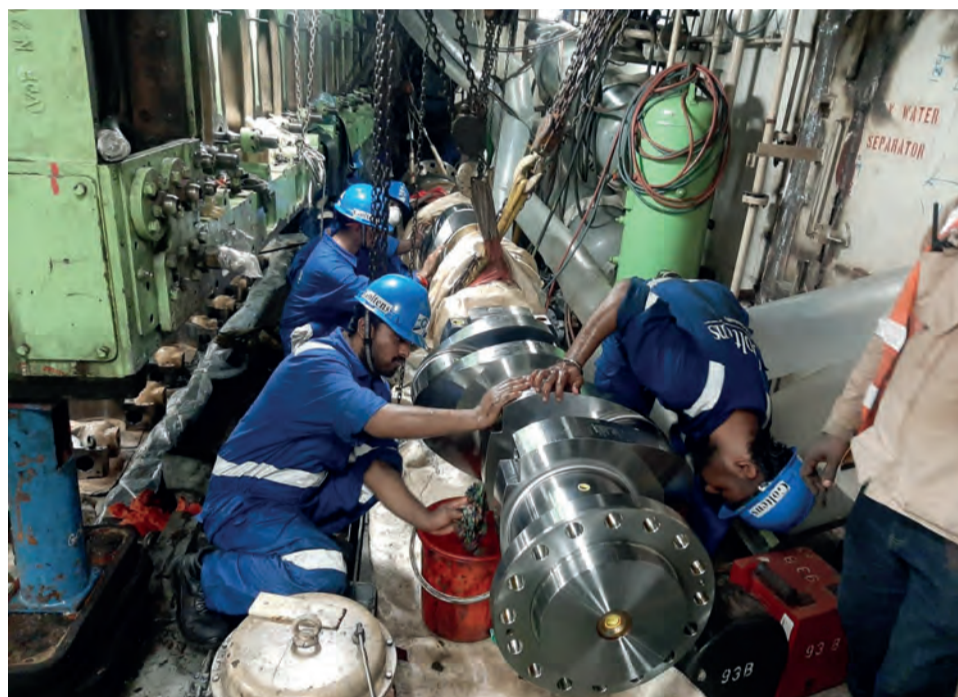
Final cleaning and inspection of new crankshaft prior to assembly
