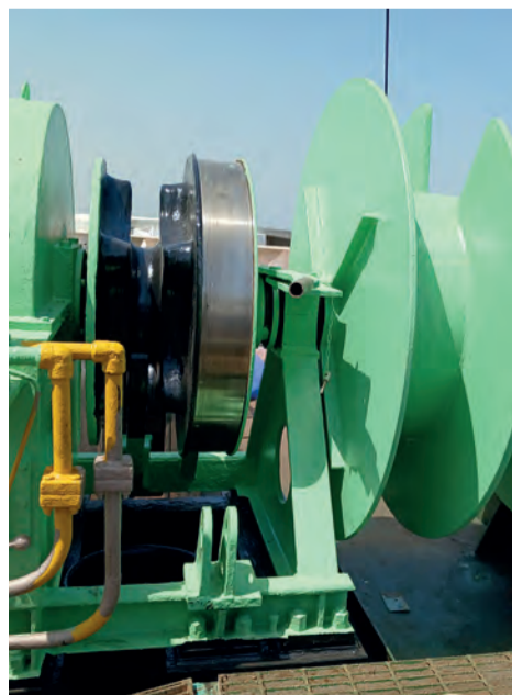
Anchor windlass after overhaul
